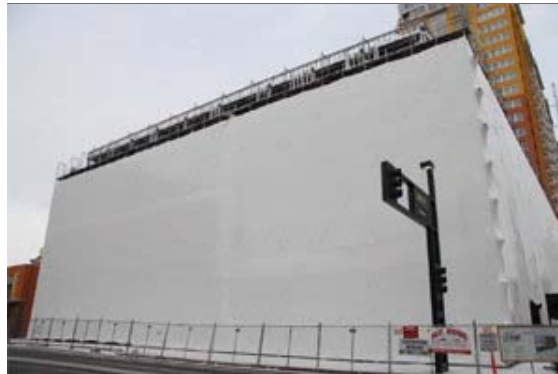
A wrapped condominium
